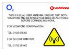
Often, additional signage may be displayed for shared antennas, such as the example here. Please ensure that the instructions are followed carefully and that both operators are contacted should the need arise.
